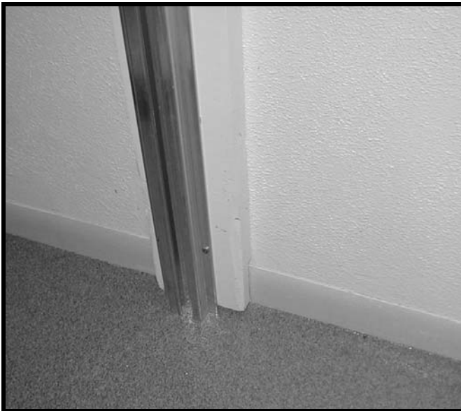
Coping the 2x6 board to accommodate baseboard.
