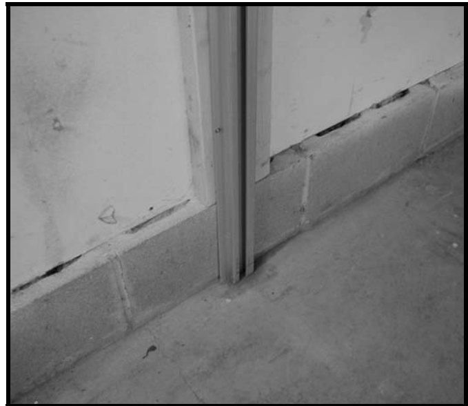
Accommodating a protruding masonry stem wall.
